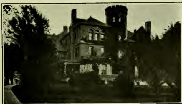
RESIDENCE OF THE LATE S. D. COYKENDALL.
